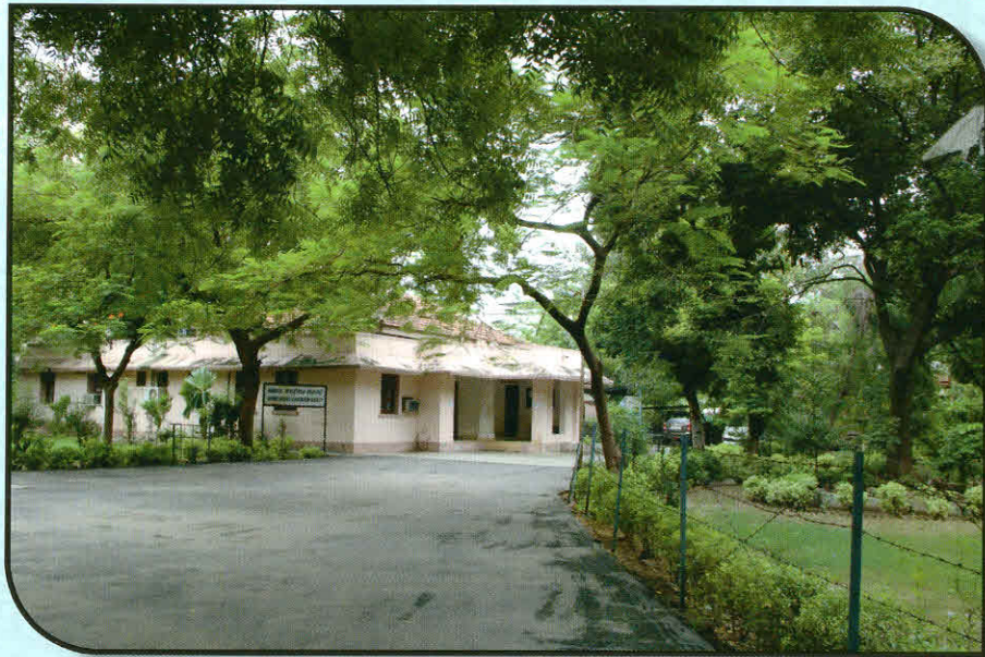
Main Office building of the Ahmedabad Education Society, Navrangpura, Ahmedabad - 380 009.
